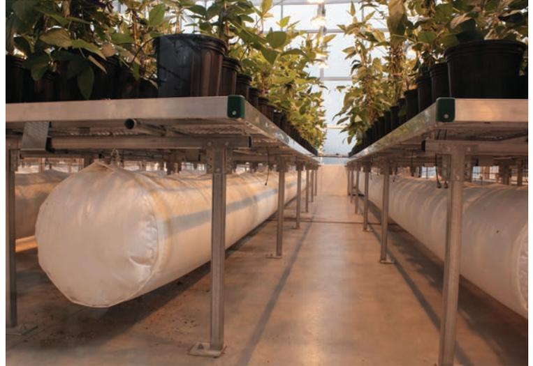
**S**ystems that utilize fabric, such as DuctSox, provide targeted, precise and efficient air dispersion for new construction and retrofit projects. Additional benefits include a total lifetime ownership cost that is significantly less than a comparable metal ductwork layout and the ability for a system to be custom designed based on the application.
