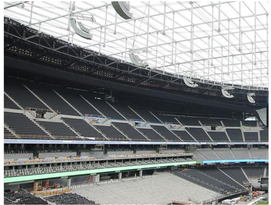
ensure a smooth transition between the ducts and scoreboards, custom “wings” were developed in a color-matched fabric from DuctSox to help retain visual consistency.
