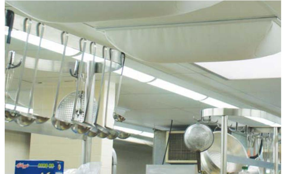
the 16-inch-high bar joists were spaced approximately three feet on center with only four inches between the bottom of the joists and the suspended ceiling. Even with proper air balance in the space, the existing conventional 2x4-foot metal ceiling diffusers presented too much draft and turbulence for exhaust hood performance.
