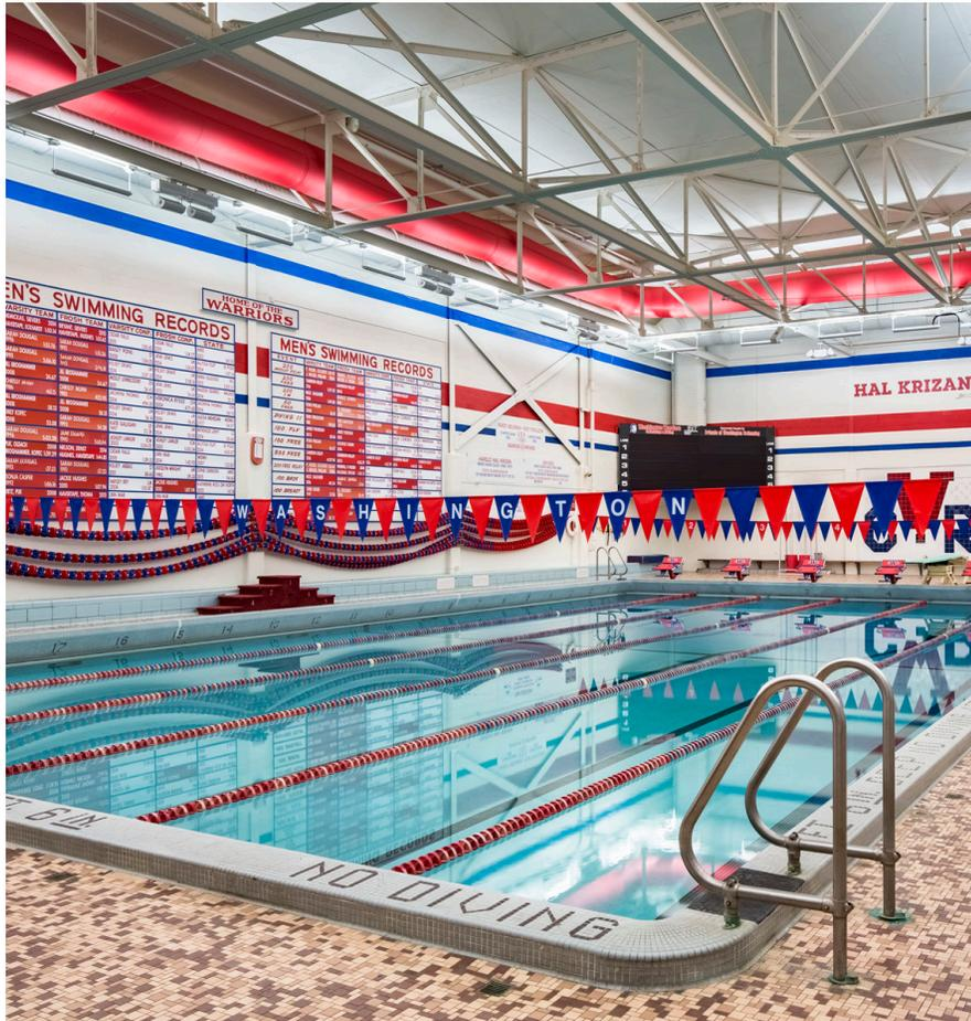
Fabric duct reduces ventilation material/installation costs and fast-tracks installation time by 60% to assure work completion during a short two-month summer recess. Shive-Hattery specifies fabric duct more frequently today, but now incorporates the industry's latest innovations such as linear L-vents for indoor air comfort, custom colors
