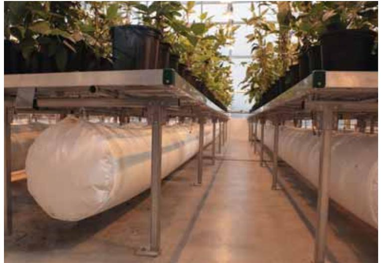
Technology advancements in fabric have created an opportunity for DuctSox to be used in applications where there are specific performance requirements. Anti-static fabrics are ideal for data centers and anti-microbial treated fabrics for laboratories, food processing and grow facilities.
